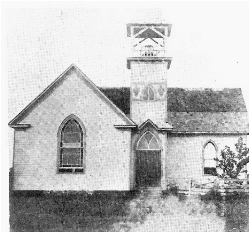
The M.E. Church, South, was originally located at 6 th and Beech. It was moved to the present location in 1923, where it became the American Legion Hall.
