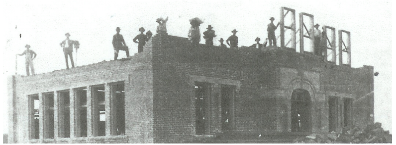
Foyil School under construction
