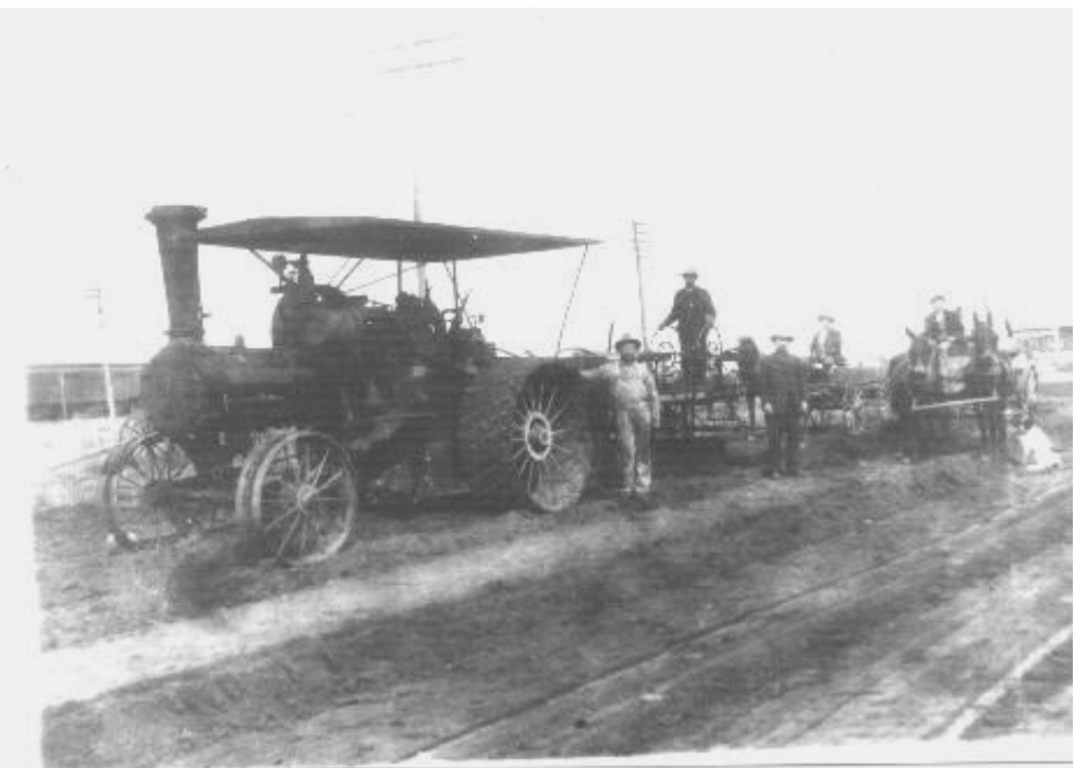
Working on the road!
