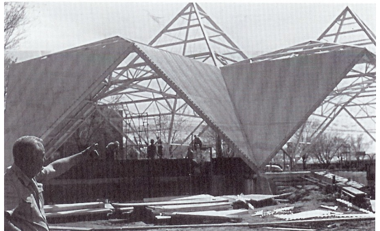
Constructing a roof over the pool in 1950 Whitaker's State Home
