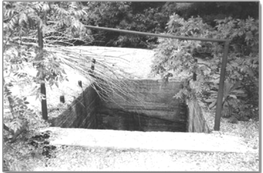
An open mineshaft in a populated part of Picher is not blocked off by any kind of barrier. Sealing it off is not among current remediation projects.
